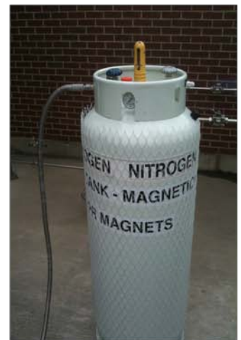
Attach fill hose to the blue liquid valve of dewar. Make sure not to overtighten the connections!!!
