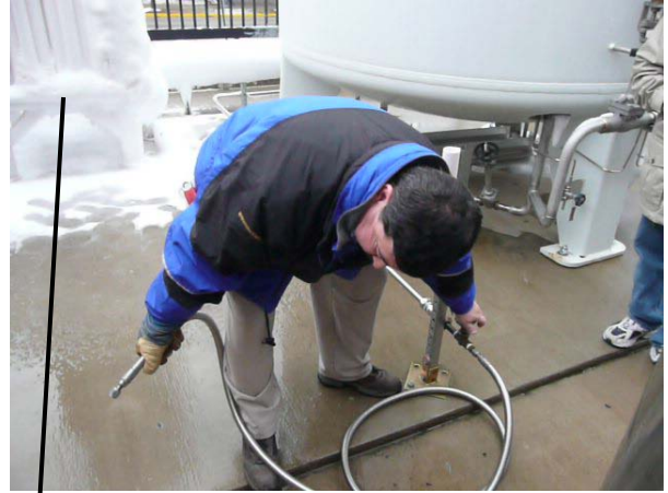
Purging the fill hose
